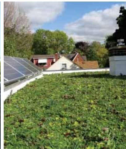
A green roof can be used to manage stormwater runoff.
