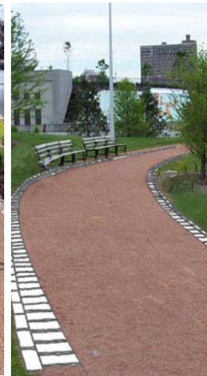
seal coat aggregate paving
